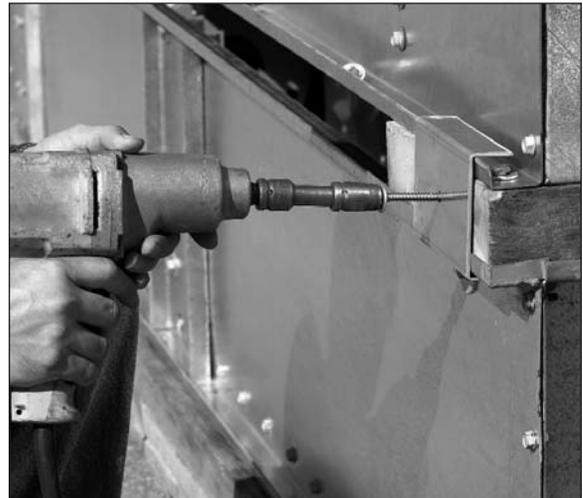
Figure 5 – Removal of shipping channels
