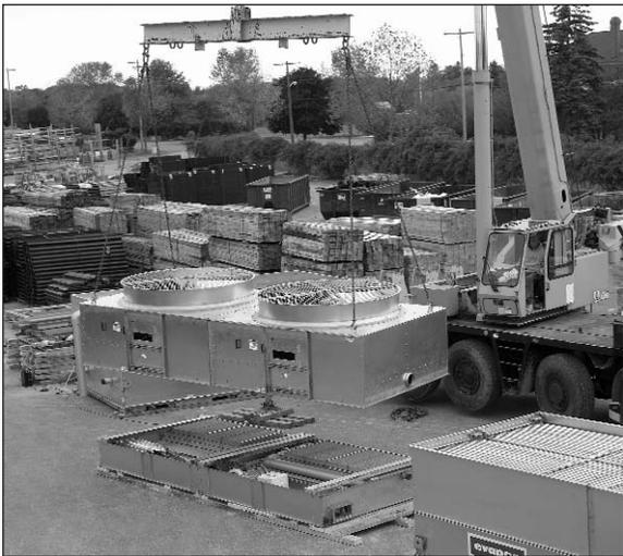
Figure 7 – Lifting of fan section
